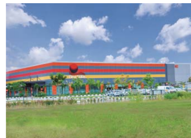
First Solar photovoltaic plant, Kulim, Malaysia
